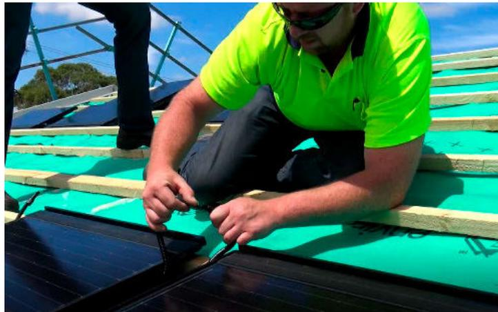
The AC wire must remain in the wire containment box of the first and last solar unit of each row. The lead connector and the same made in situ, are fitted in flexible and solid HD conduits between the isolator and the first and last modules to complete the circuit.
